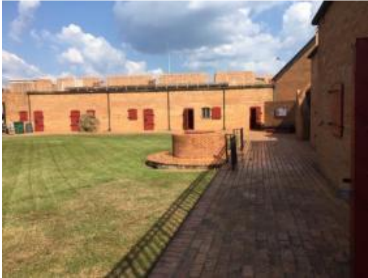
Portion of interior courtyard
